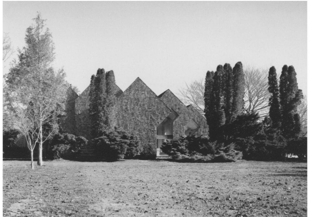
Anteroom with view westwards | View from the west showing the series of pointed gables
