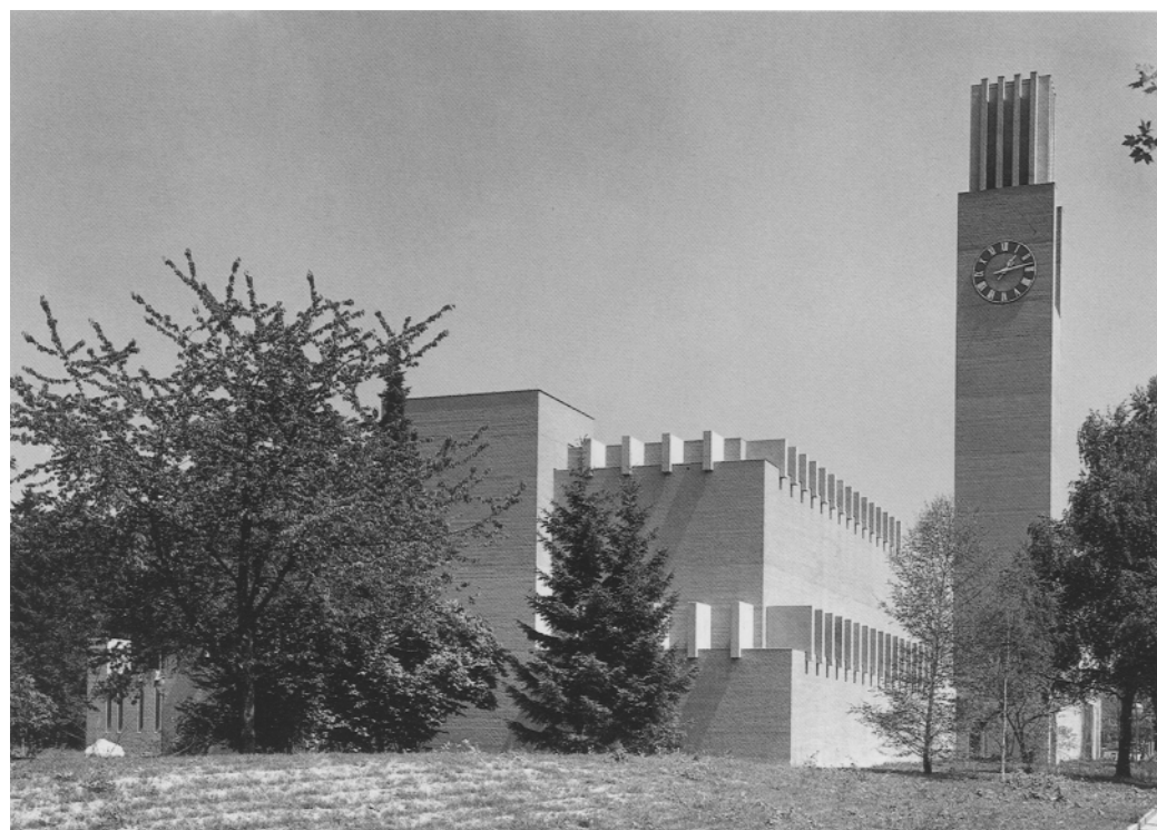
Churchyard with the base of the tower on the left, in the background the entrance to the church with the cast aluminium panels of the relief "Water and Fire" by Bernard Schorderet | View from the west with the 35 metre high "campanile" | Main church showing the combined altar, pulpit and font, hung below the rooflight the wall tapestry by Moik Schiele | Back of the church hall with the musicians' gallery
