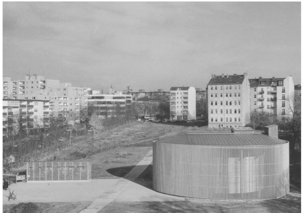
Entrance from outside | Chapel on the strip of the former Berlin Wall, with the path formerly used by the soldier patrols running through the centre, view northeast | Interior with the altar on the left and retable saved from the demolished Church of Reconciliation in the niche on the right | Ambulatory between the outer and inner skin, on the left the door to the chapel
