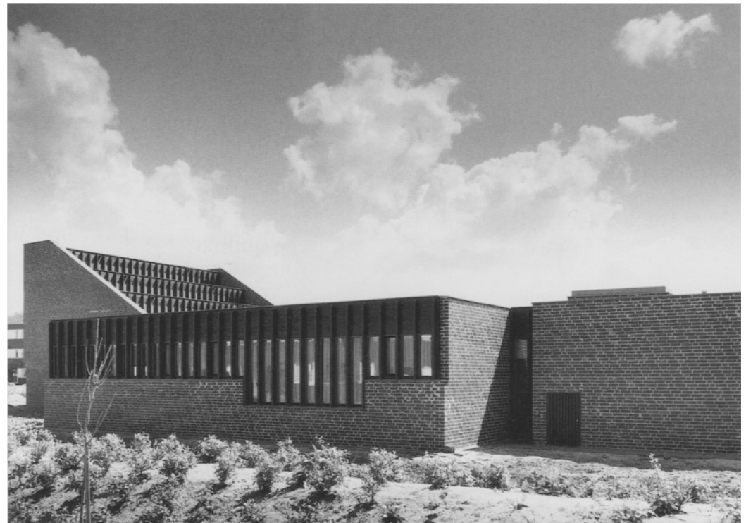
View from the southeast, entrance in the background | View from the northwest, in front the row of windows of the youth centre, behind the stepped roof of the nave | Parish hall, in the top centre the opening for the bells | Internal courtyard looking to the southwest, youth centre in the background | Nave of the main church with fourfold stepped skylight, right the transition to the parish hall, left the vertical shaft with the bells
