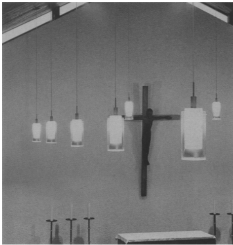
8 Karl Hans Neumann, Church of St Joseph, Müncheningen, 1962 Diffuse light: a translucent inner cylinder containing an economical compact fluorescent lamp produces diffuse ambient lighting for daytime church services
