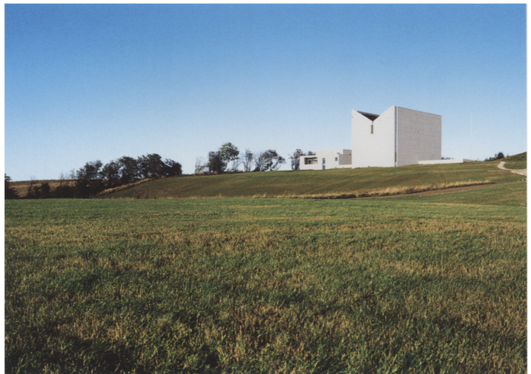
View of the church and ancillary buildings from the southeast | View from the west | Kneeling rest and altar, behind them the backlit wall niche | The stringent processional arrangement of the church is even reflected in the material joins
