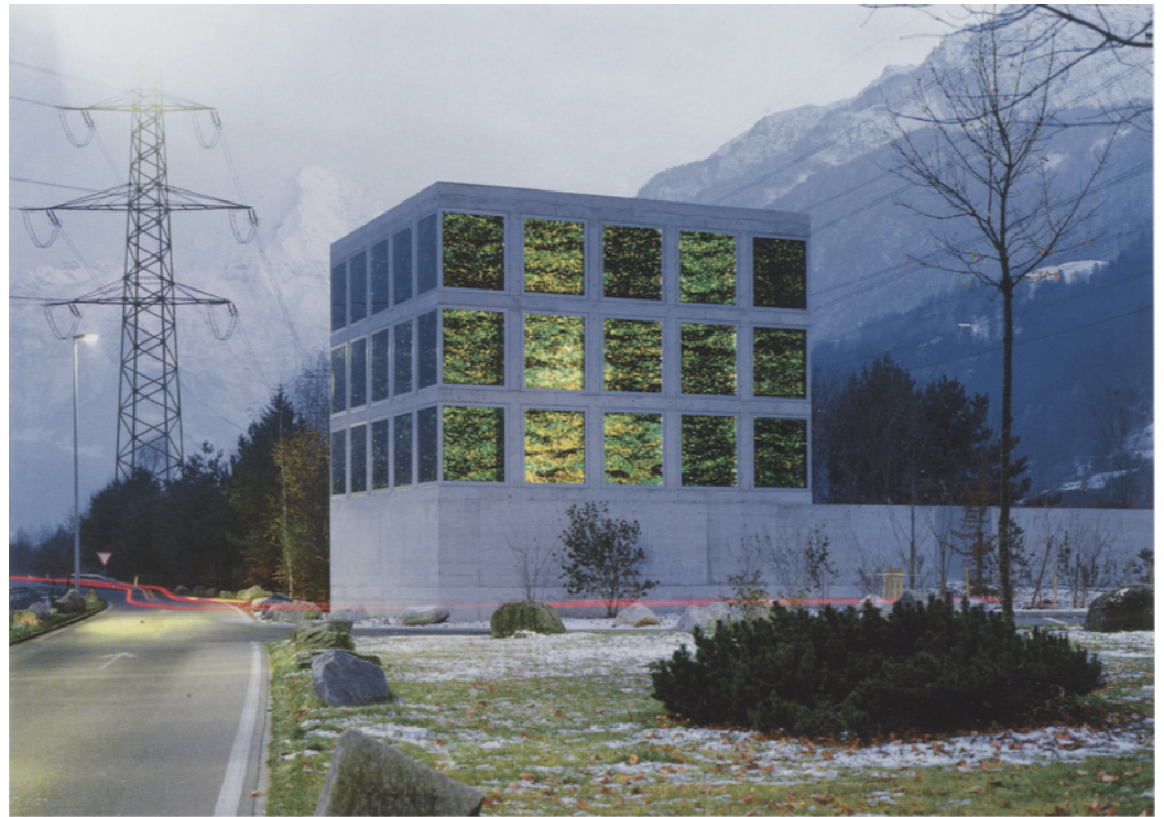
View from the west over the courtyard and building, aluminium-framed windows extend around all four sides of the frameless box | The cuboid of the chapel seen at dusk illuminated from within
