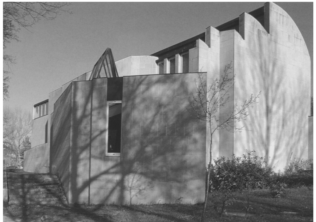
View from the east, left the wing with offices and hall | View from the northwest, baptistry to the front | Nave with the rounded arches in reinforced concrete | View from the gallery onto the side entrance and the transition to the sacristy
