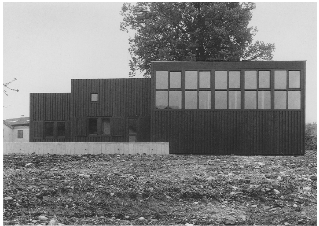
View from the south | View from the north, left the seating wall | Part of the "entrance hall" with way through to the church space | View from the hall looking west, above right the mullioned windows
