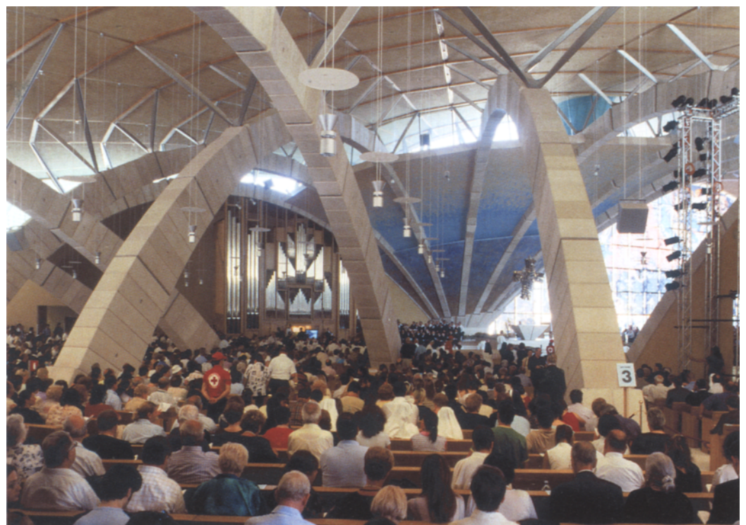
West entrance in front of the axis from the baptistry to presbytery, to the right the bronze doors by Mimmo Paladino | View of the altar and organ, lighting from the large window on the right and from rooflights between the roof sections | The arcs of the arches with segments of five or six blocks each, top left a V-shaped steel supporting strut for the roof rests at the intersection between two segments of the arch
