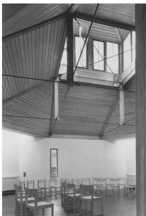
View from the east, at the rear the canopy of the multi-purpose space | Main building from the upper level with corner tower and central tower, entrance to the vestibule on the left | View from the southeast, on the left the house, on the right the church, in the centre the narrow window level with the hall | Way through from the vestibule to the hall, in the corner, rear right, one of the four small obscured rooflights | Visible transparent construction of the roof, which additionally subdivides the plain space of the hall
