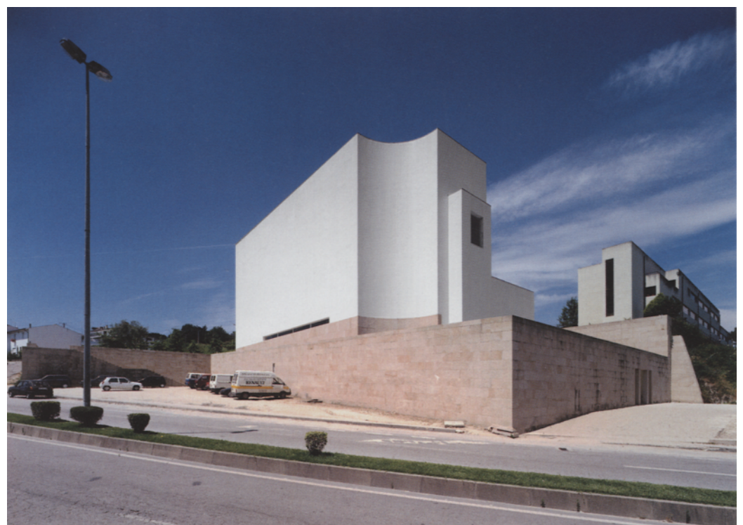
View from the southwest, to the left the "tower" with the baptistry, to the right the "tower" with the weekday entrance and belfry | View from the east, plinth clad in granite, to the right the entrance to the lobby of the funeral chapel
