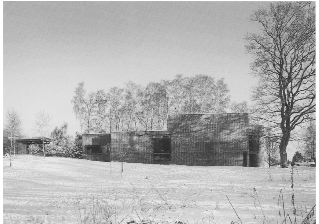
The church hall from the east, clear glass mounted in black steel frames | View from the west, right the high space of the church, left the low canopy
