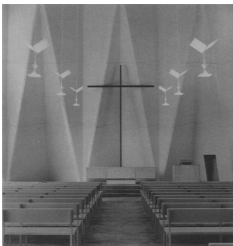
9 Maier Graf Speidel, Grace Church, Stuttgart, 1964 Soft light: the winged light fittings echo the folds in the concrete ceiling and walls. The matt glass and white perforated metal sheets reflect the light from the lamp producing a soft light within the church interior
