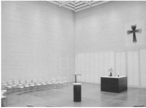
4 Florian Nagler, St Sophia, Munich, 2005 White timber slatted screens filter natural light that shines from above and through the rear wall. The mean daylight factor lies between 5.7 and 6.4 per cent
